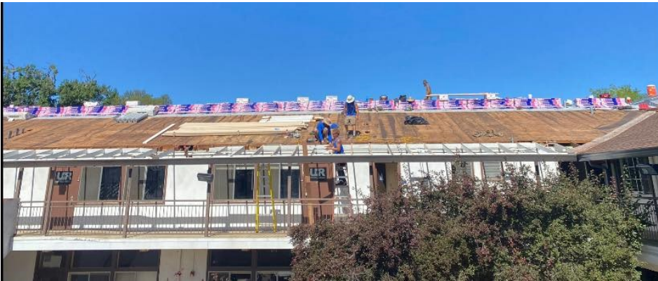
Repairing the dry rot in the overhang outside Room 209.
