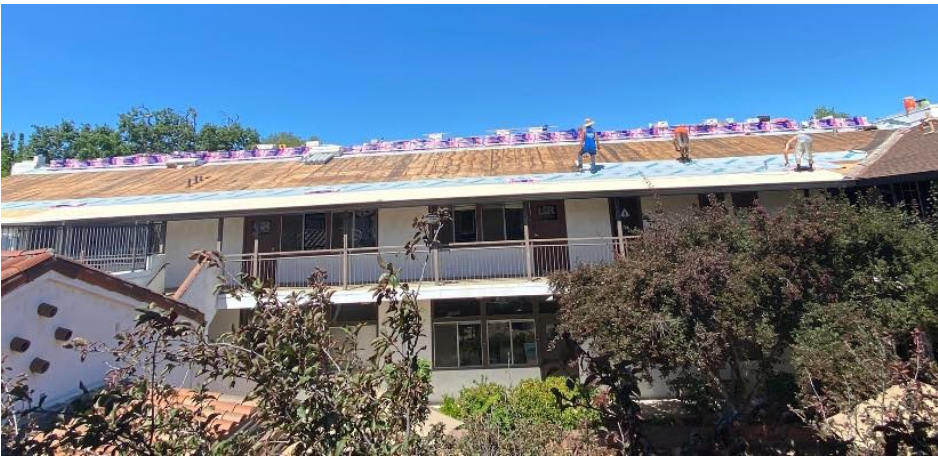
Installing the underlayment in preparation for shingles
